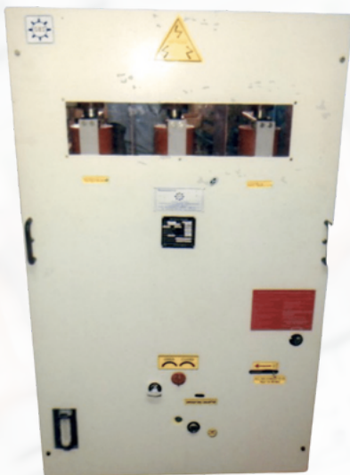
Retrofitting VCB Suitable for Easun 22 KV
